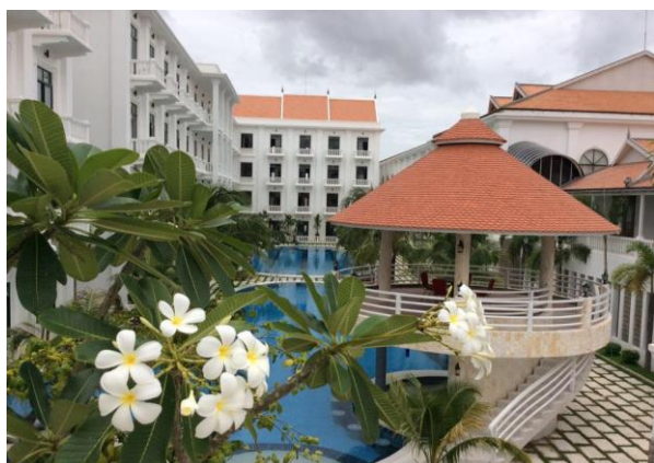
View of the main building from front side
